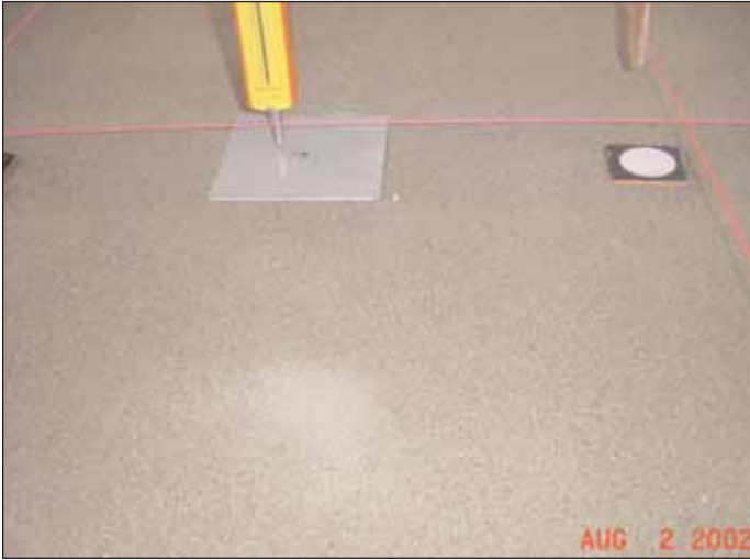
Hair Crack Behind Reinforced Zone after First Shaking Load Application
