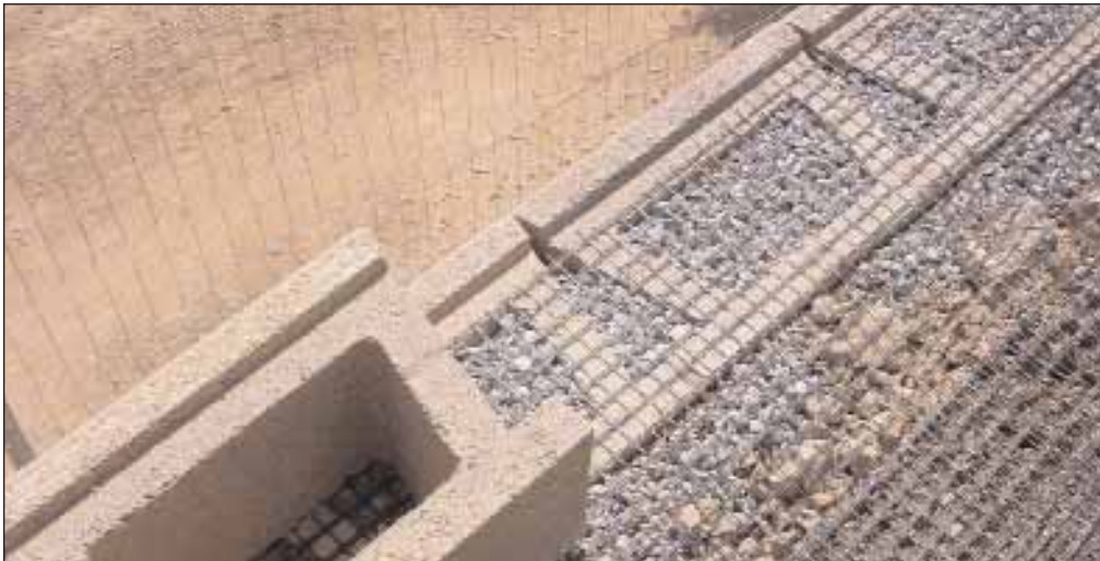
Allan Block reinforced with Huesker geogrid.
